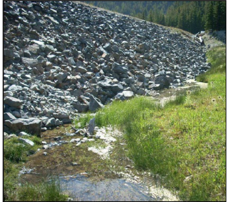
Figure 1: Seepage Emanating from Downstream Toe of Embankment Dam (Photo Courtesy of the Department of Natural Resources and Conservation)
